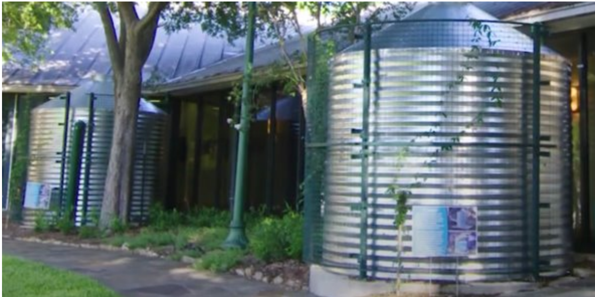
Figure 9 - An example of a roof-gutter-downspout-cistern system.
